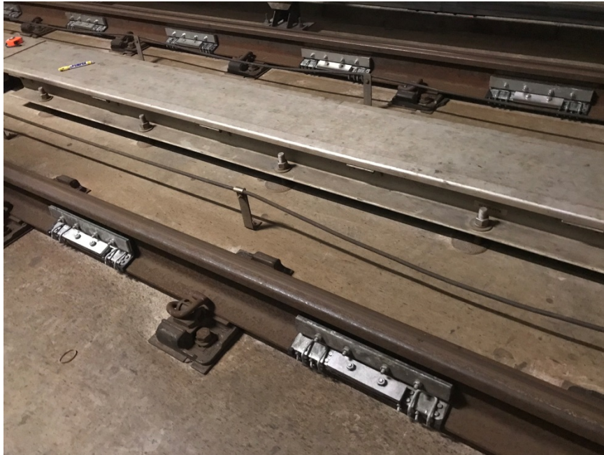
Figure 4 Track with rail dampers installed
